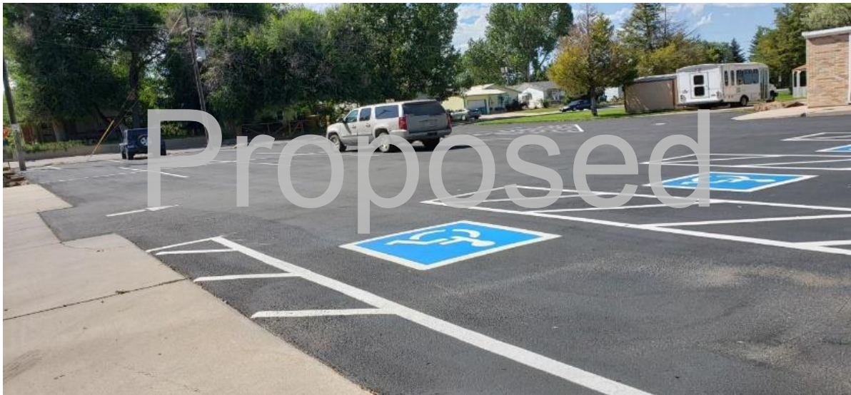
Example of seal coat/ crack fill project
