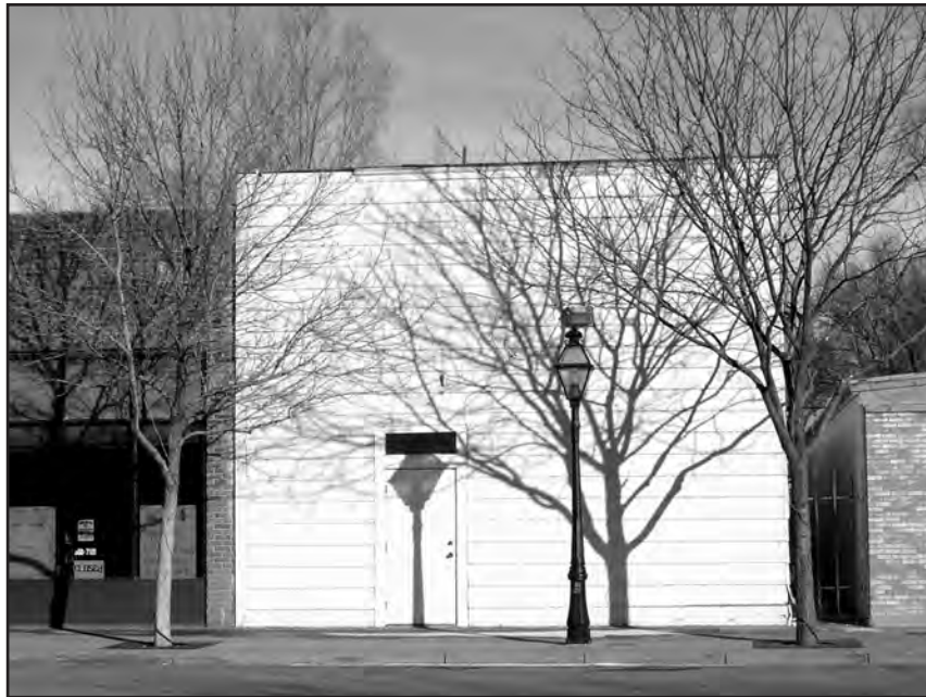
3740 Cleveland Avenue before renovation - 2004
