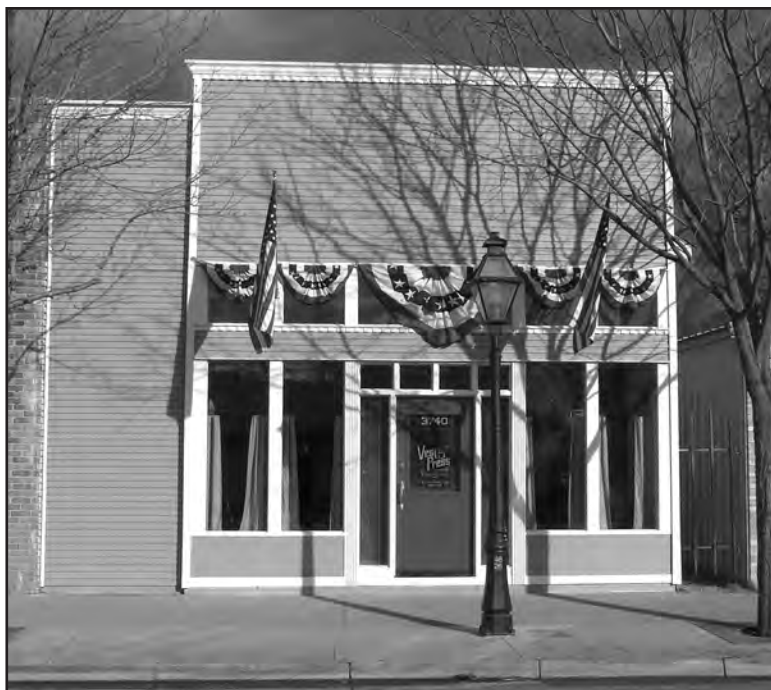
3740 Cleveland Avenue after renovation - 2005
