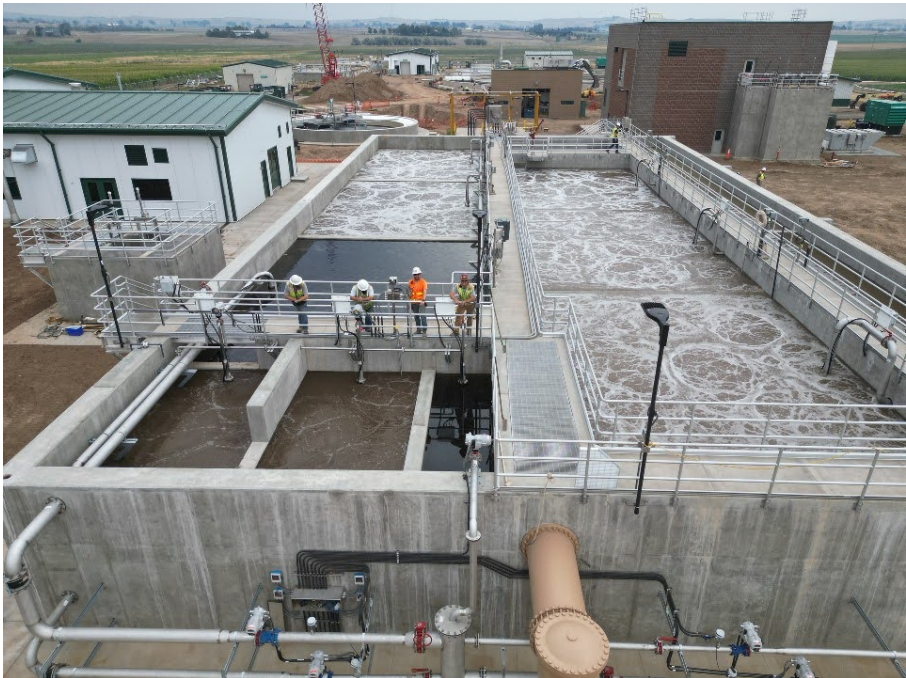
Photo of the Water Reclamation Facility just prior to substantial completion.
