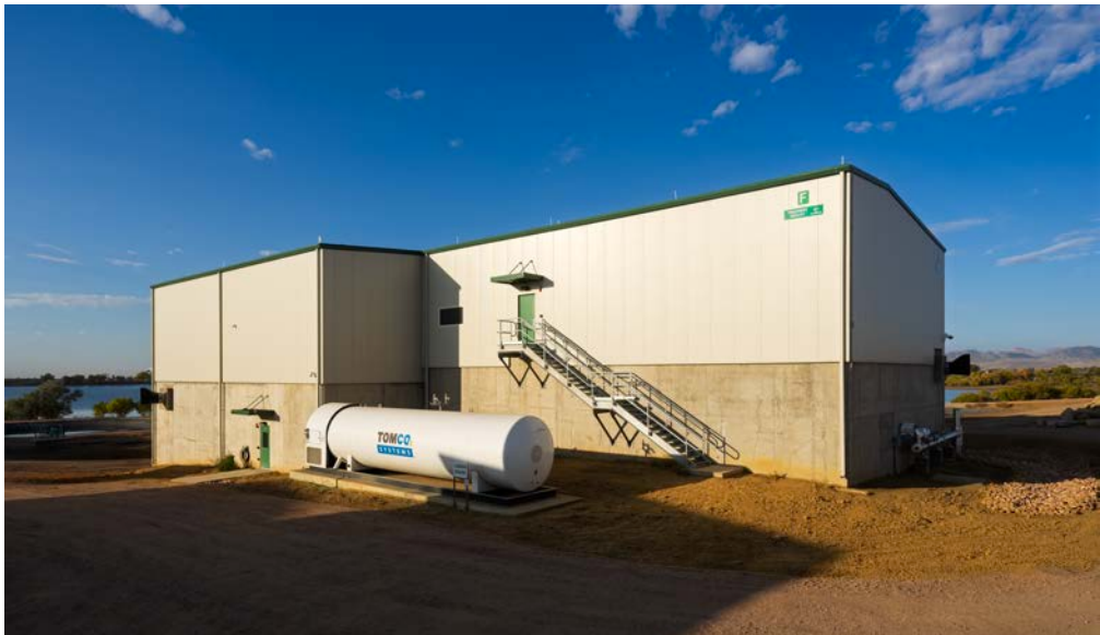
Photo of the newly expanded Water Treatment Plant.
